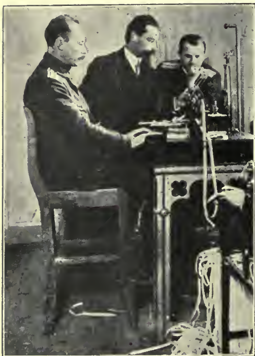
OFFICE OF THE BREST-PETROGRAD DIRECT TELEGRAPH IN THE CONFERENCE BUILDING.
