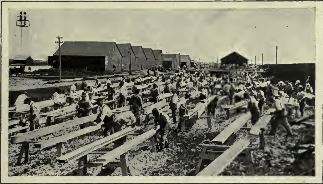
BUILDING AN AVIATION CAMP, JULY, 1917.
