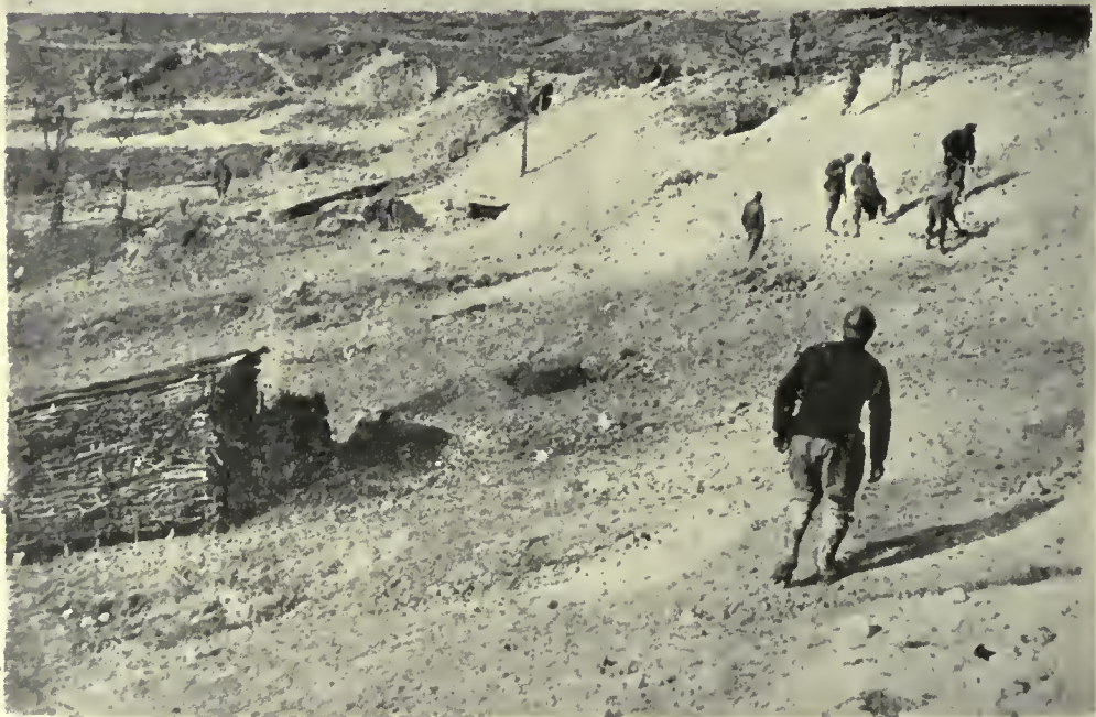
REPAIRING UNDERGROUND SHELTERS AFTER THEIR CAPTURE.
