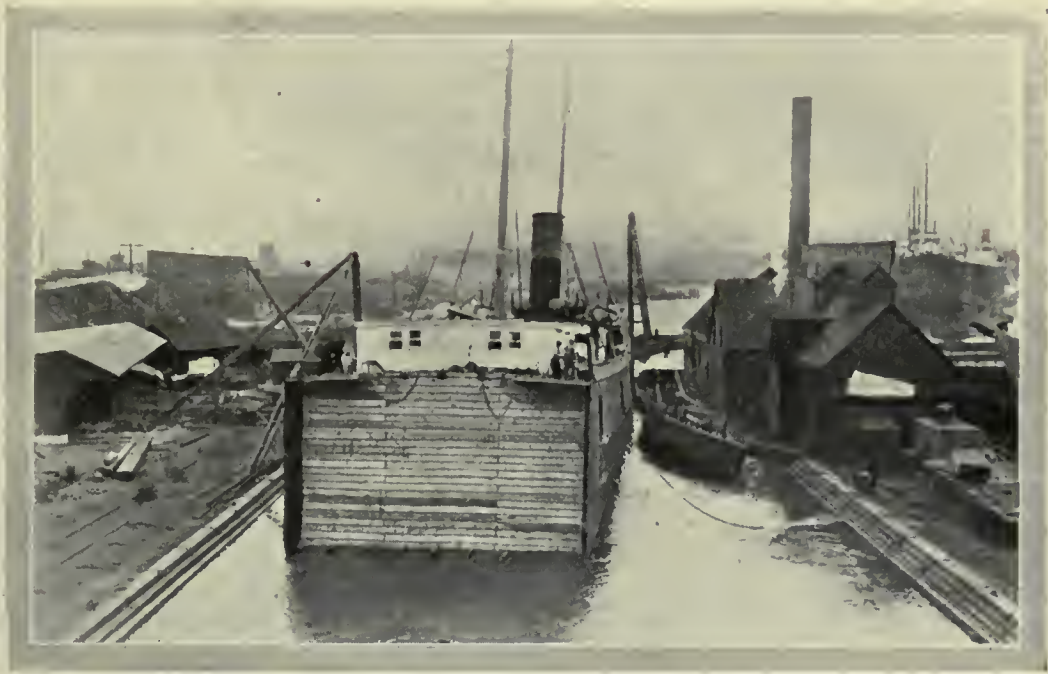
THE STERN PORTION OF THE SAME STEAMER ON ITS PASSAGE TO THE COAST, WHERE THE TWO HALVES WERE REASSEMBLED.
