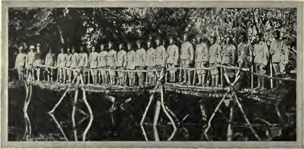
SAPPERS OF THE WEST AFRICAN REGIMENT (Sierra Leone) ON A BRIDGE OF THEIR OWN CONSTRUCTION.
